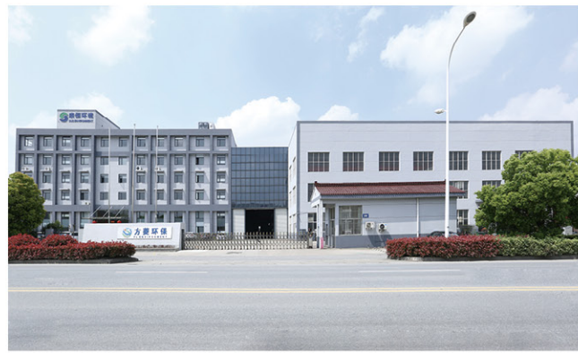
Wuxi Manufacturing Plant (Phase I)
